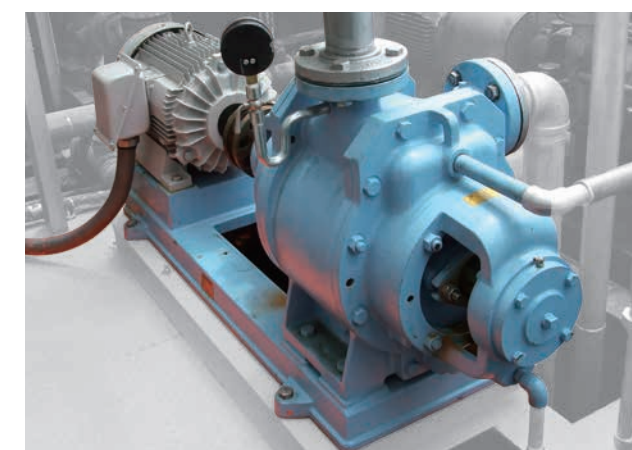
Bag Filter for Fly Ash Handling Vacuum Pump 65V611, 11 kW × 1150 min -1 5.5 m 3 /min × -500 mmHg (G)
