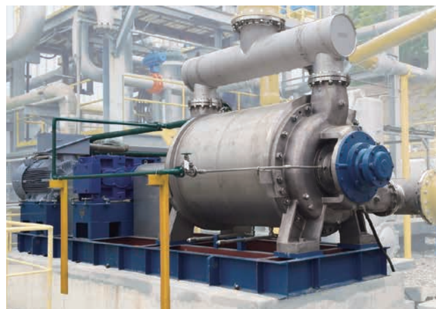
Vacuum Pump for Condenser Gas Extraction System 250VL4280G, 280 kW × 275 min -1 184 m 3 /min × 33.6 kPa (abs)
